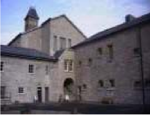
Ruthin Gaol Grade 1 Listed Building. Work included lime pointing to all stonework
